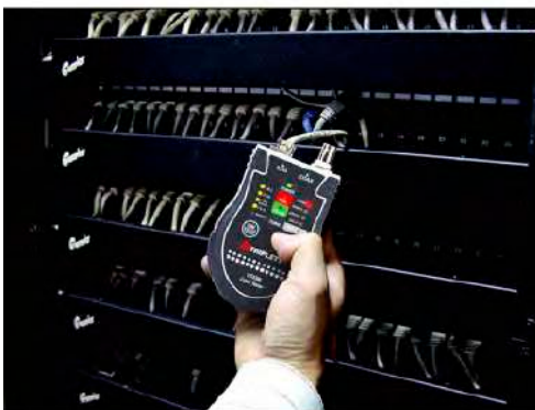
Confirm continuity and fault type
